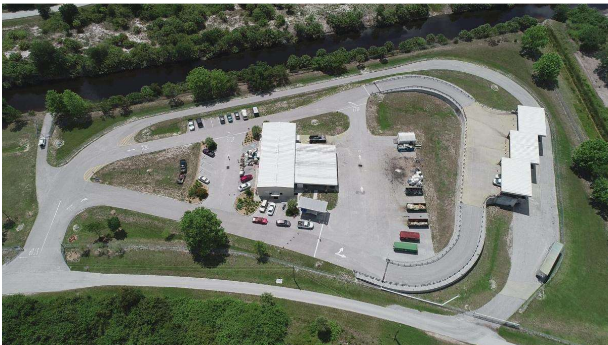
Figure 3 - A hybrid below-ground / ground-level direct-to-bin transfer station
