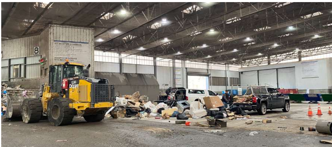
Figure 4 - Example of a tipping floor
